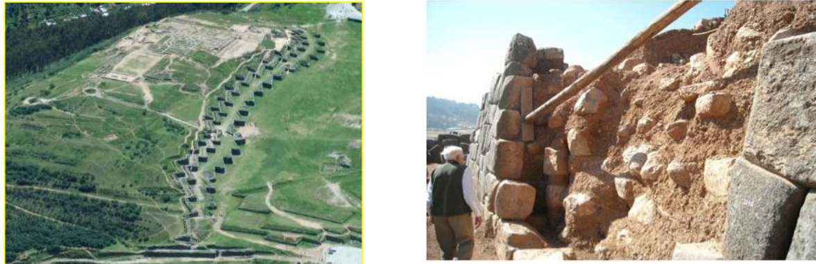
Figure 1. View of Saqsaywaman Park (left). Collapsed Inca wall (right). (Miksad et al., 2013)
